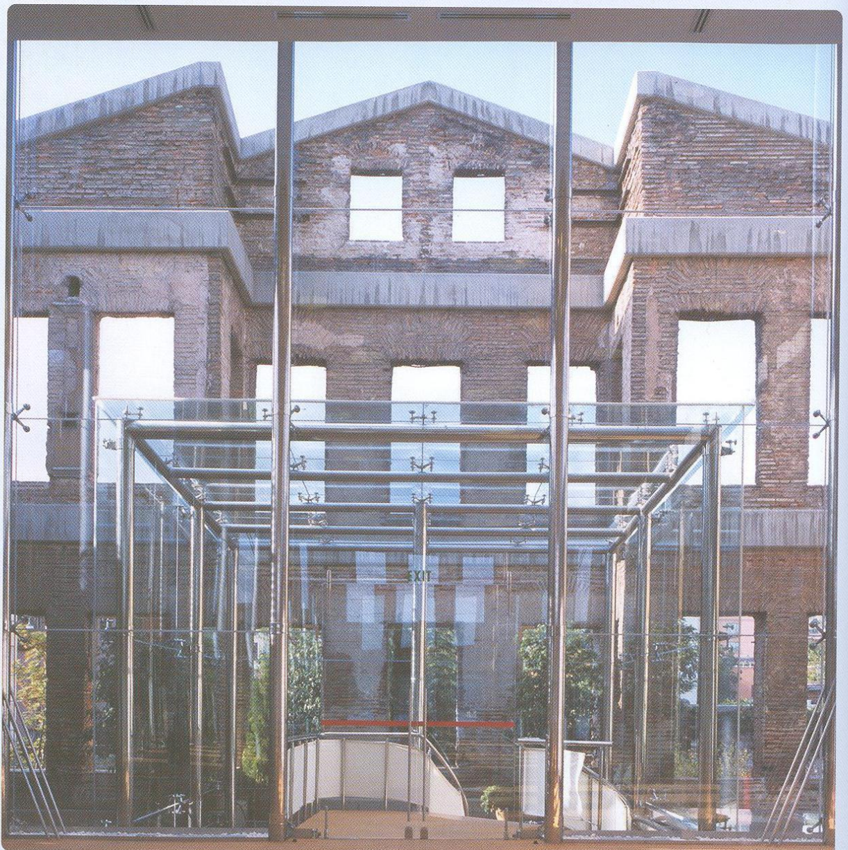
Gökhan Avcıoğlu, Philippe Robert and Haluk Sezgin, Adaptive reuse of 200-year-old Esmâ Sultan Waterfront House, Istanbul, 1999 Top and bottom A glass box with a frameless suspended glass system is constructed inside the remaining historical walls in order to prevent the new intervention from overshadowing the old building.
